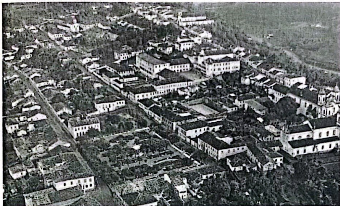
Figure 26 – The low central area with Gomes Freire square in the foreground
