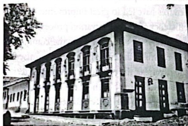
Figure 16 – Private buildings in need of restoration around Gomes Freire square
